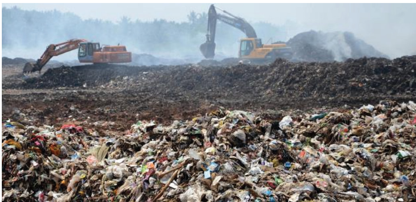
A Coimbatore Landfill: Contractor appointed to manage waste is non-compliant with guidelines regarding safe waste disposal
