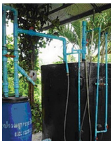
Generation of methane/bio-gas in bio- digester
