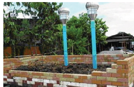
Open air composting with air vents and drainage pipes
