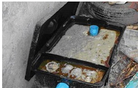
Grease traps installed at households
